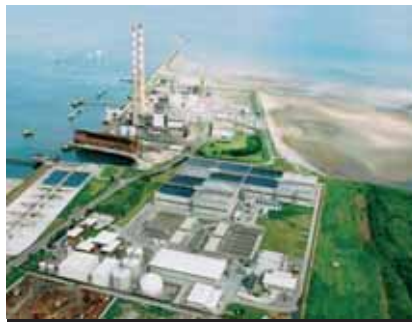
Dublin Bay Wastewater Treatment Works
