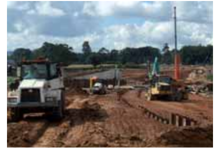
Norton Fitzwarren Dam under construction
